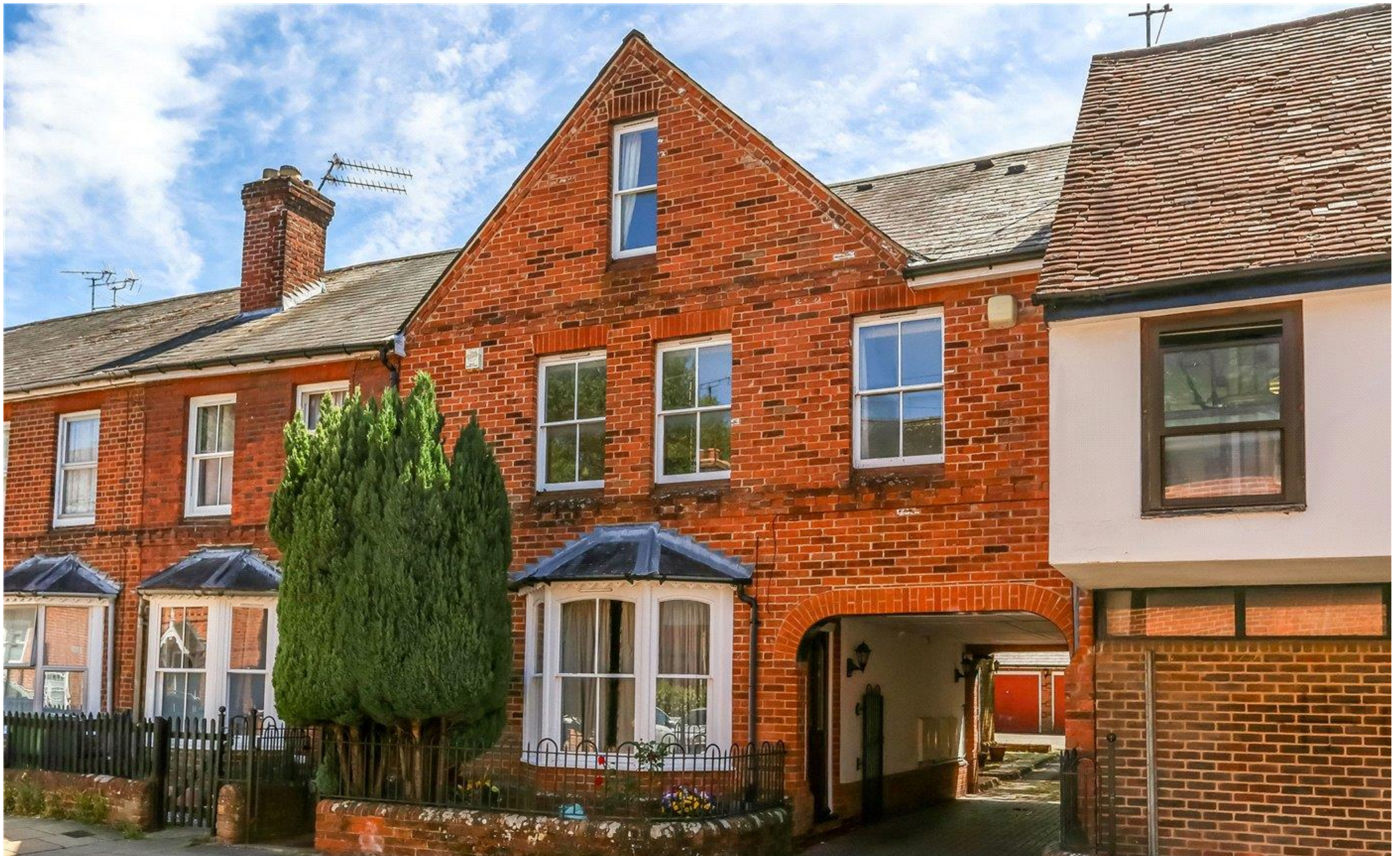
Old Bakery Yard, Middle Brook Street, Winchester, SO23 8DQ
