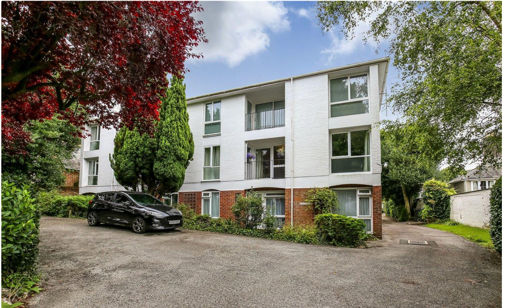
Fairlawn House, 11 Christchurch Road, Winchester, SO23 9SR
